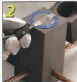
2 Attach control unit termination clip to ignition strip
