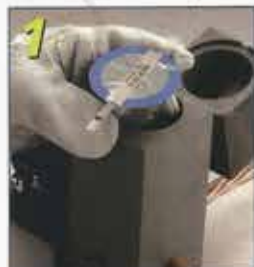
1 Insert CADWELD® PLUS package into mould
